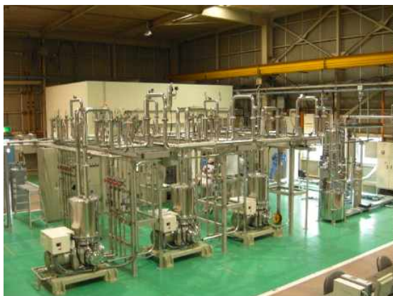
Fig. 3. Cooling system used at the Asahi power station managed by TEPCO. Circulating LN2 temperature: 66 K - 80 K, Cooling power: 5 kW @ 70 K, Flow: 30 L - 60 L/min, ΔP: 250 kPa.
