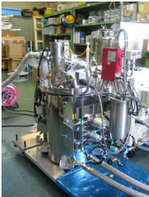
Fig. 4. He gas circulation cooling system for NMR sample cryo-probe. Operation temperature: <20 K, Mass flow: 0.1 g/s, Cooling power: 3 W.
