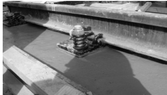
(b) Anti-vibration Clamping Device
