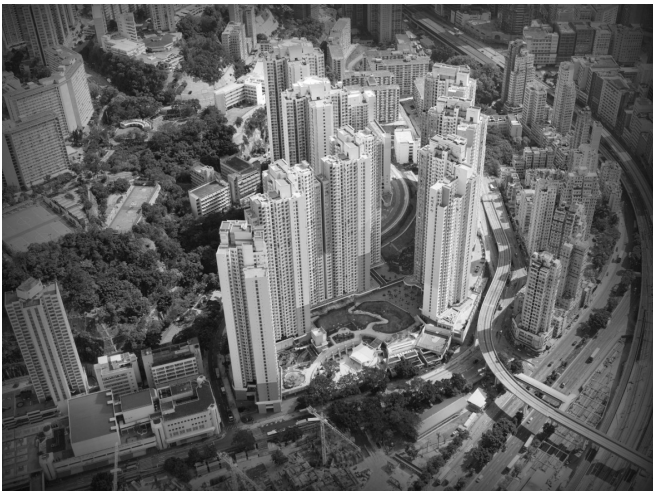
Fig. 8. Redevelopment of Upper Ngau Tau Kok Estate
