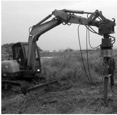
(a) Construction equipment
