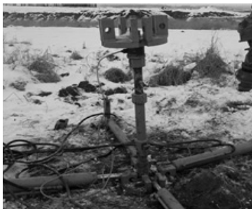
(a) Installation of hydraulic cylinder and central shaft
