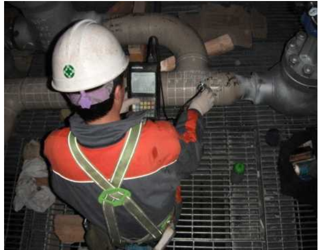
Fig. 2. UT inspection.
