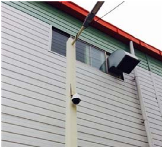
Fig. 5 Installation camera on solar street lights
