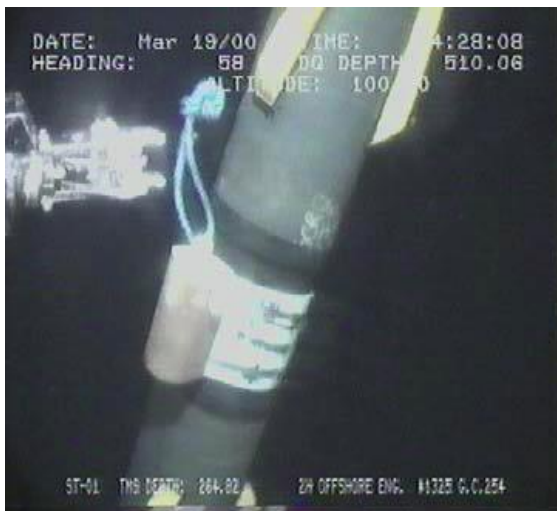
Figure 4. Installation of a subsea data logger system on a riser using a remotely operated vehicle..
