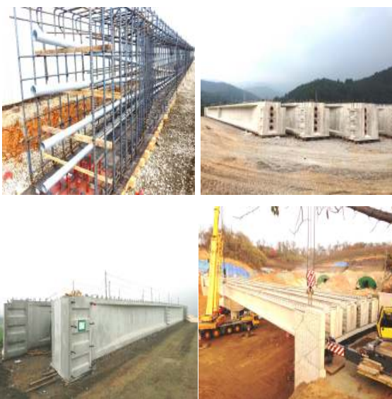
Fig. 10 B.I.B Girder Work Flow
