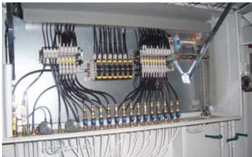
Figure 1: Central system for hydraulic controller
