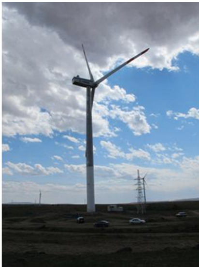
Fig. 7. Grid-connected trial operating of the 3.6MW half direct-driven wind power generator with immersion evaporative cooling system
