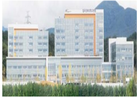
Fig 1. The complete view of the subject building
