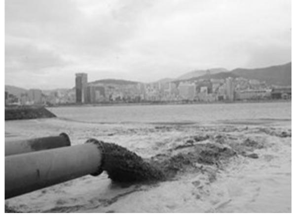
(b) Outlet from pipe in Pusan port
