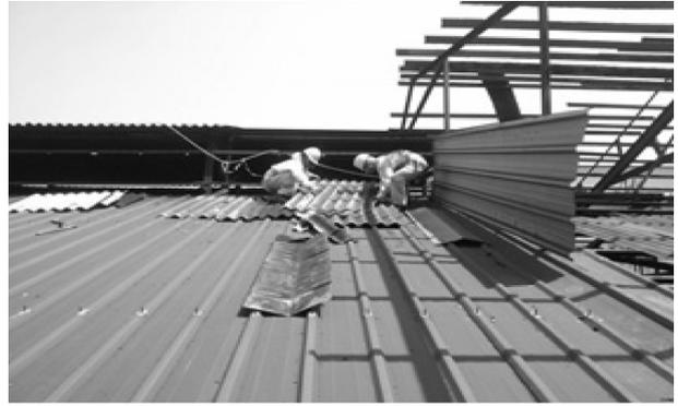
Fig. 1. Removal work of the asbestos cement slates.
