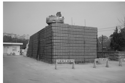
(h) Construction completed
