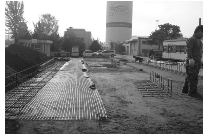
(b) Install primary reinforcement
