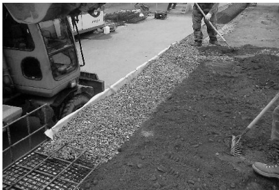
(e) Backfill gravel
