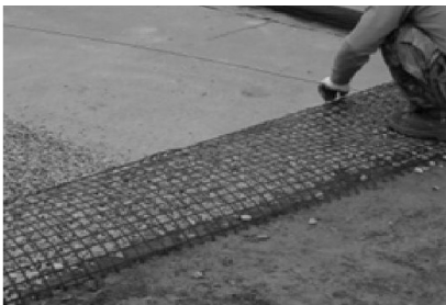
(g) Roll reinforcement
