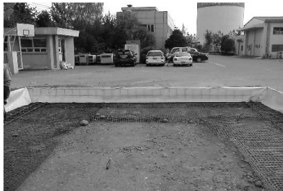
(c) Install secondary reinforcement
