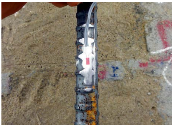
Fig. 5 Steel Strain Gauges Installation on the Longitudinal Steel (Detail)
