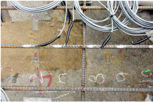
Fig. 2 Steel Strain Gauges Installation on the Longitudinal Steel (Detail)
