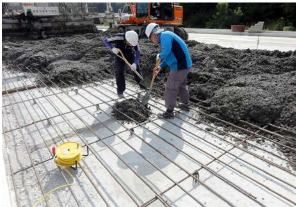
Fig. 8 Concrete Pouring at Steel Strain Gauge Location
