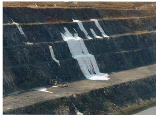
Fig. 5. Groundwater flow vestige at the Gyeongyangcheon cross-section.
