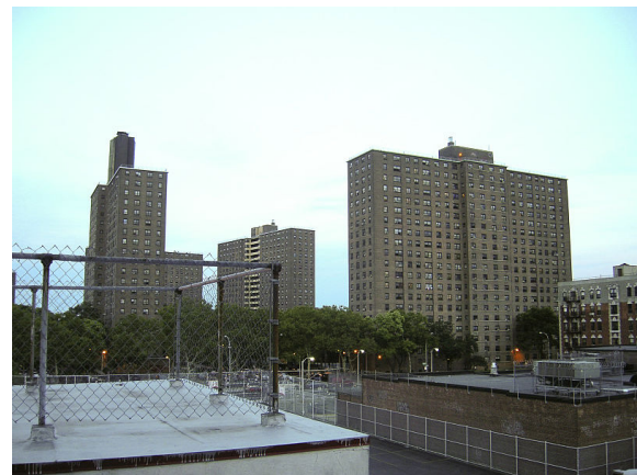
Figure 1. The 20-story John F. Hylan houses in the Bushwick section of Brooklyn, New York City
