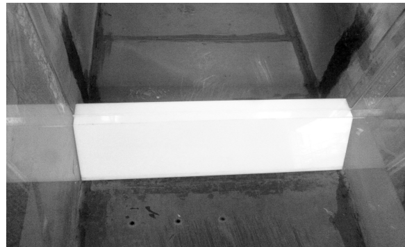
(b) Photo of Overflow Type Weir Installation
