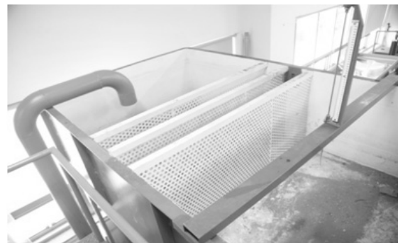
(b) Rectification Wall Installation in the Channel of Controlling Discharge
