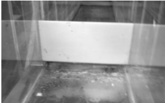
(a) Photo of Underflow Type Weir Installation
