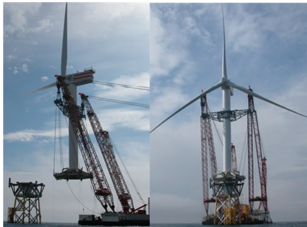
그림 2 The Rambiz installing a fully assembled turbine at Beatrice ( http://www.scaldis-smc.com/beatricewindfarm.html )
