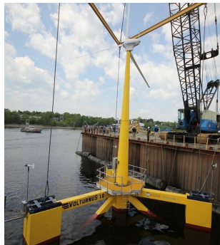
Fig. 5 VoltturnUS: Scaled pilot floating wind turbine of DeepCwind project (20kW)
