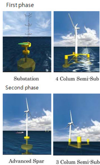
Fig. 6 Platforms for Fukushima floating wind farm
