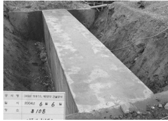
(b) Reinforcement by connection beam
