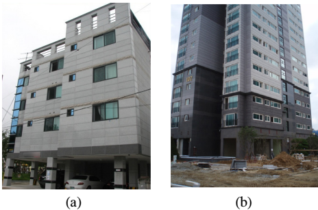
[Fig. 1] Piloti-type RC Shear Wall Structures (a) low-rise building (b) High-rise building
