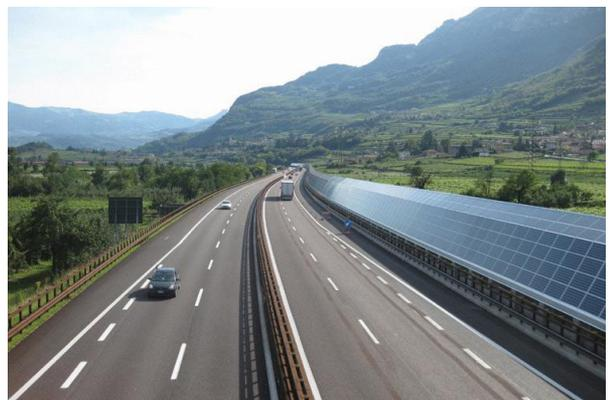
Fig. 3 Photovoltaic Soundproof Wall in Italy
