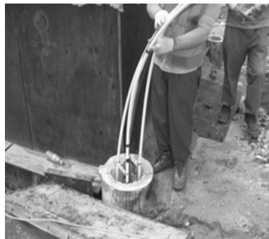
(b) Installation of GHE into piles
