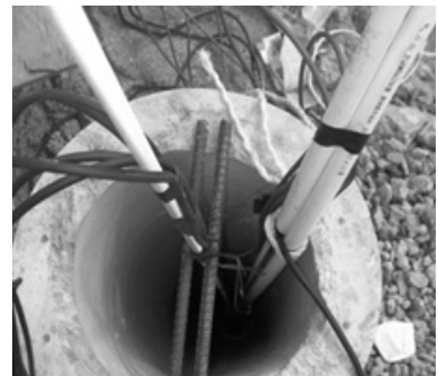
(c) Attachment of sensors
