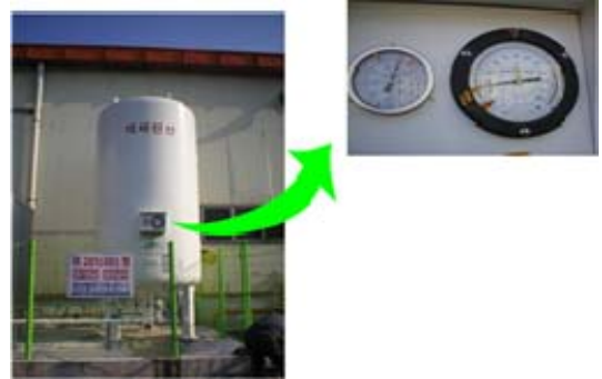
Figure 1: Analog Liquid gas level gauge
