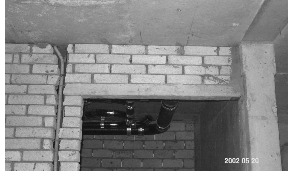
<Figure 3> Reinforced concrete lintel beam
