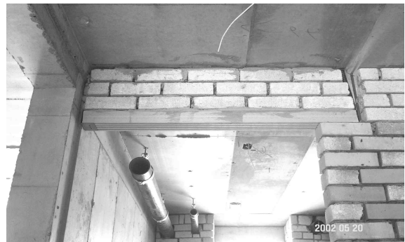
<Figure 4> Extruded lintel beam
