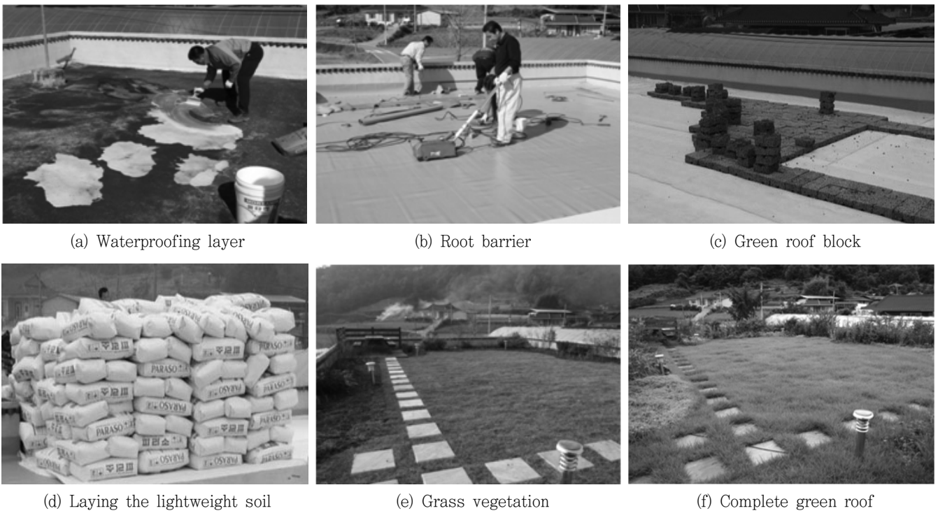
Fig. 2 Process of green roof construction
