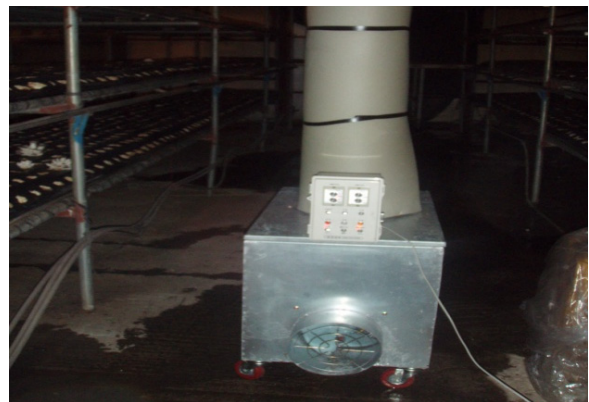
Figure 3. Air circulation unit setting in the oyster mushroom farm.
