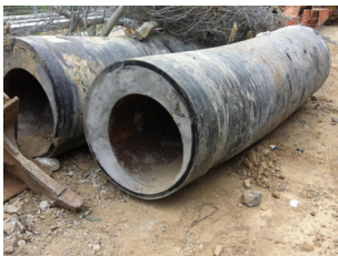
[Fig. 6] Bowed drainpipe(PE double wall pipe)
