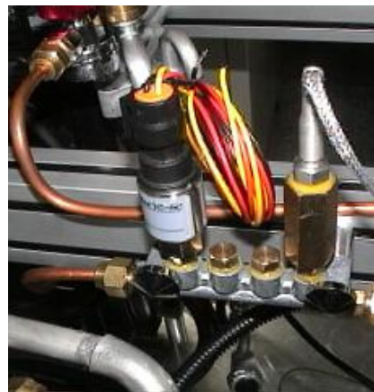
[Fig. 4] Pressure and Temperature Sensors
