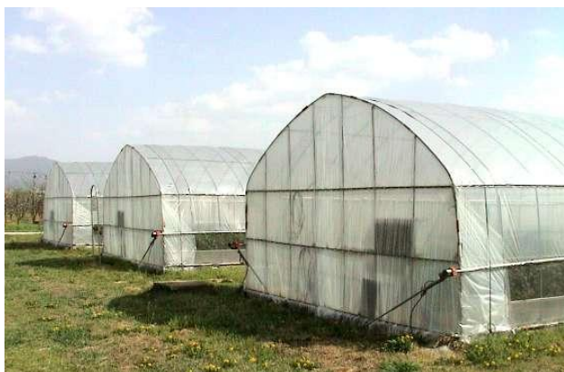
Figure 1. Quonset Greenhouse with Polyethylene film
