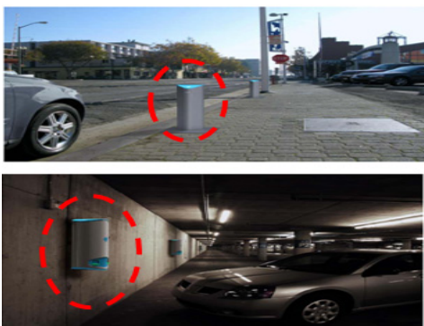
[Fig. 3] Wireless Charger in Parking
