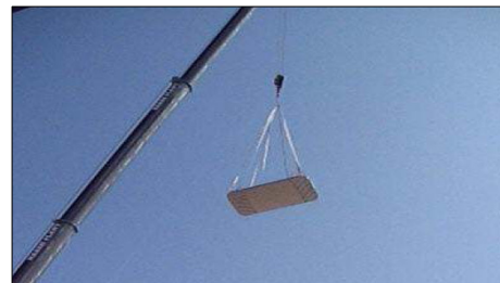
[Fig. 9] 65ft Lifting of Fuel Cell
