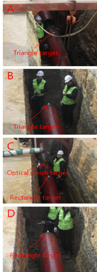
Figure 7. Underground facilities surveying using targets
