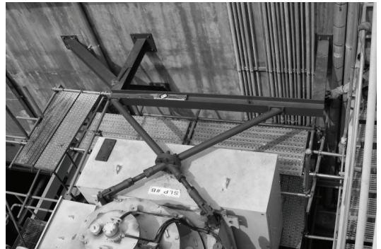
Fig. 13 Picture taken for the actual machine modified with stiffeners
