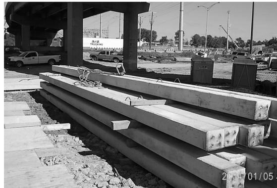
Fig. 4. Rectangular prestressed pile (Application case in USA AASHTO(2007))
