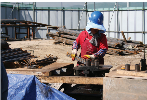
Figure 5. Factory processing of rebar
