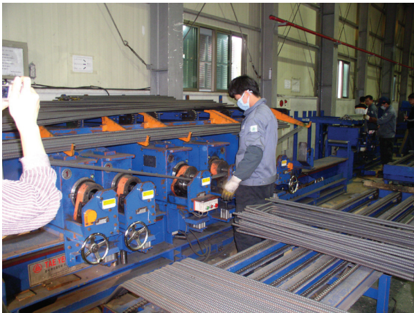
Figure 4. Field processing of rebar
