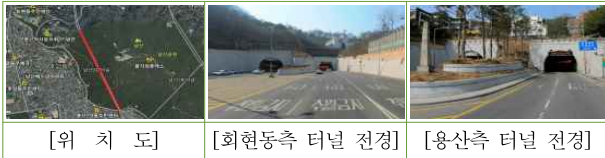
〈Figure 7〉 Location and foreground of Namsan No.3 tunnel
