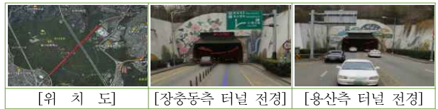
〈Figure 4〉 Location and foreground of Namsan No.2 tunnel
