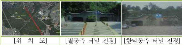
〈Figure 1〉 Location and foreground of Namsan No.1 tunnel
