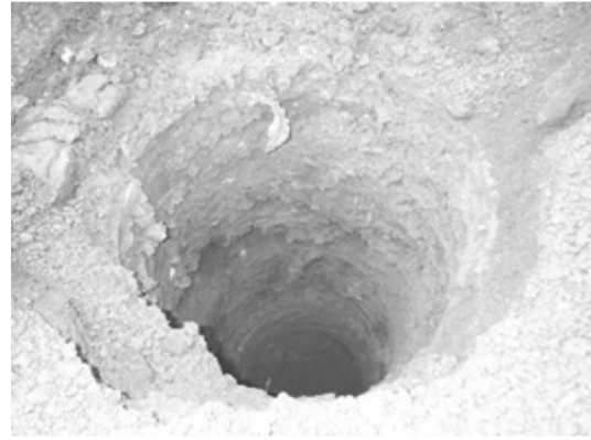
(b) Excavated hole for a foundation
