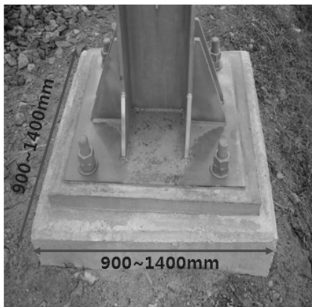
(a) Rectangular concrete foundation
