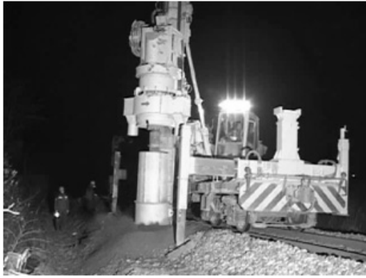
(a) Boring machine operating on railroad
