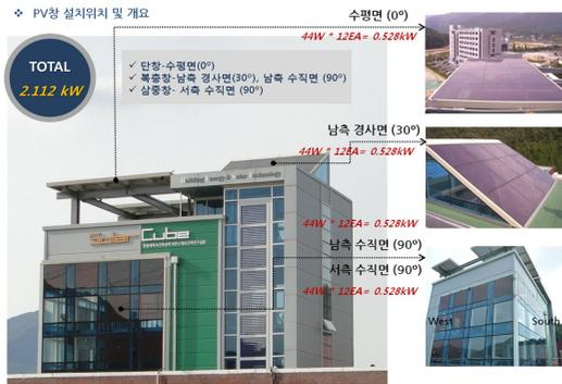
Fig. 3 Mock-up view and position of PV window
