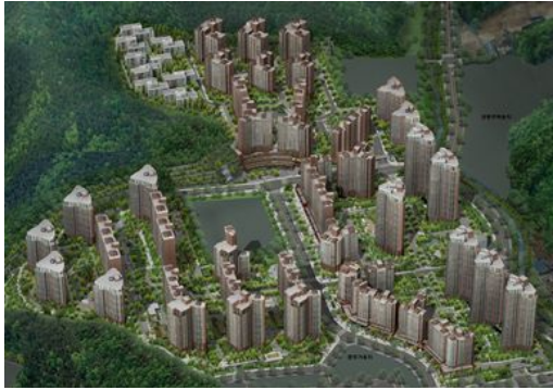
Fig. 1 Site bird view
