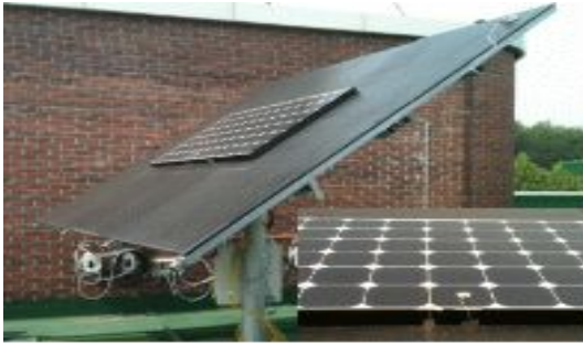
Fig. 4 PV module installation with Roof-attached type
