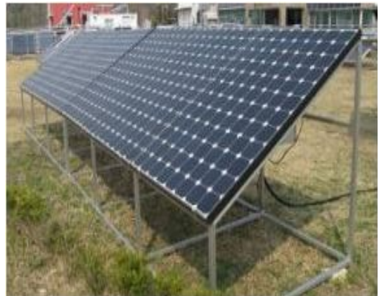
Fig. 1 PV module installation example with open-rack structure
