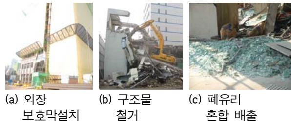
Fig.2 Deconstruction of office building
