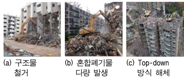
Fig.3 Deconstruction of apartment houses
