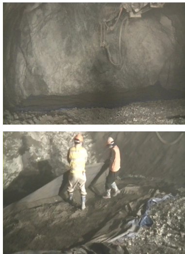
Fig. 6 Rebound test of shotcrete
