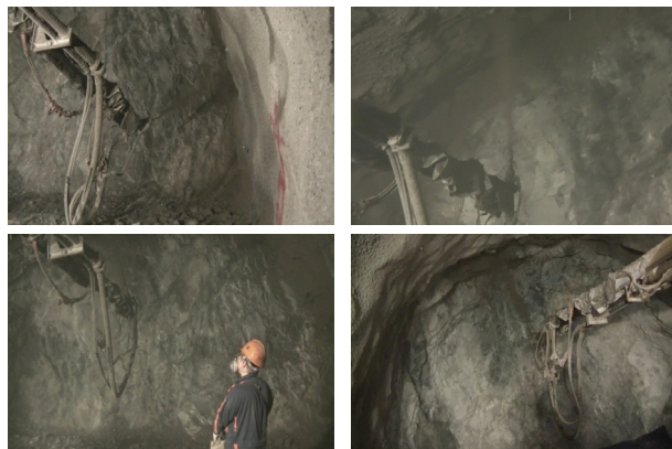
Fig. 7 Whole views of experimental construction for polyamide fiber reinforced shotcrete
