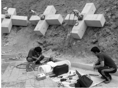
(a) Initial jacking of anchor
