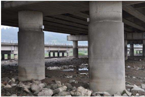
Fig. 2. Concrete cover condition after 3 years of CP construction.
