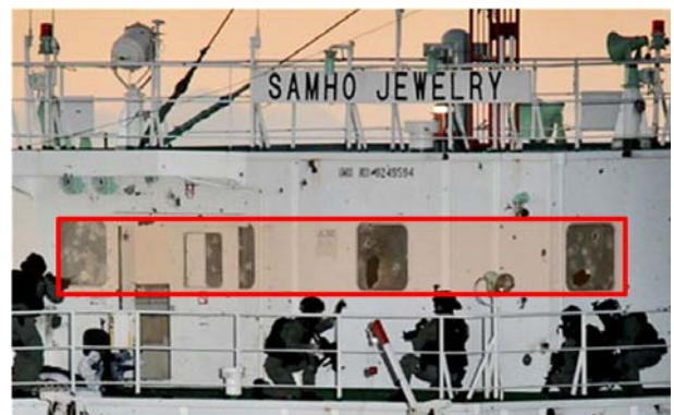
Fig. 9 Weak point of bridge (M/V Samho Jewelry)
