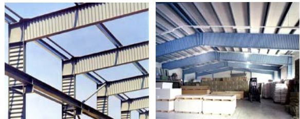
〈Fig. 1〉 Portal frame and Corrugated web
