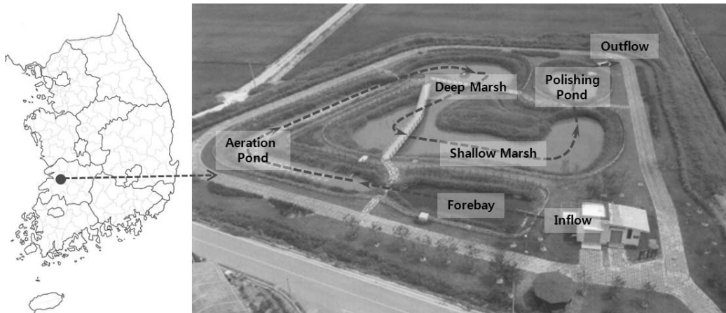
Fig.1 Location of stormwater wetland used for this study and its elements
